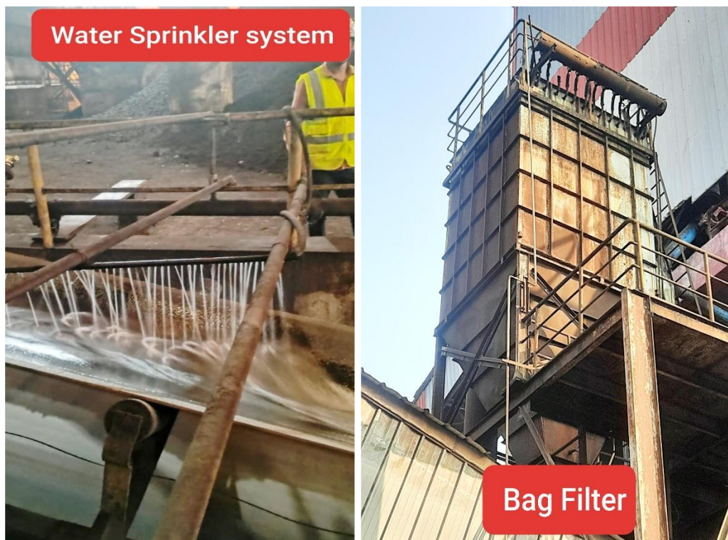
Photograph of the Water Sprinkler System and Bag filter
